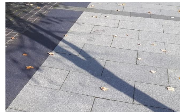
Concrete flags – granite effect
