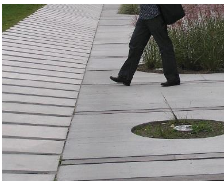
Brushed concrete footpath
