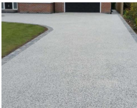
Bonded gravel path
