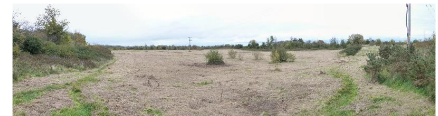
4. View from SW corner across site
